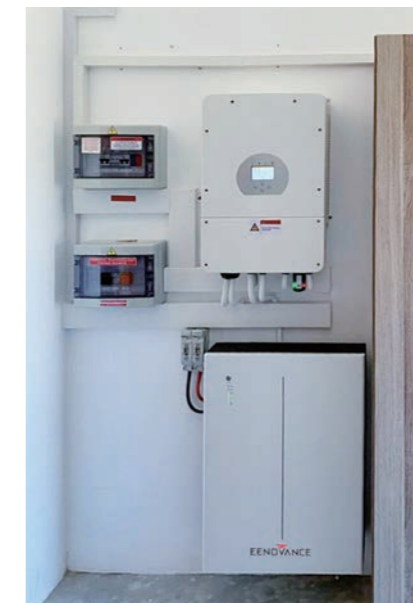
10.65kWh ● July, 2025 ● Location: South Africa ■ Configuration: MANA 10.6 battery
