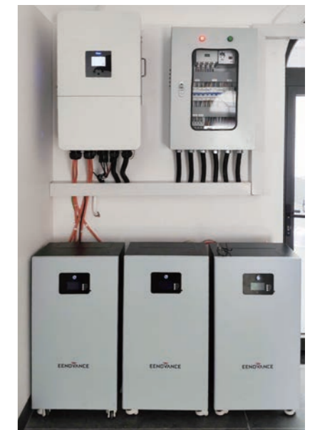
48.21kWh ● September, 2025 ● Location: Vietnam ■ Configuration: 3 * MANA 16.0 batteries
